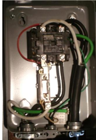
Step 8: If a voltage reading of 220 volts is present on the output legs (Fig. 5), check the wire connections on the motor starter box. If no problem is found have the motor starter box checked by your local electrician.
